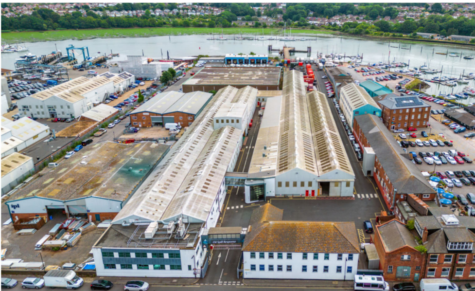
Figure 2 - Marine and Industrial businesses by the River Itchen in Northam
